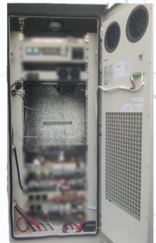
C-DOT BBU in ODU Chassis
